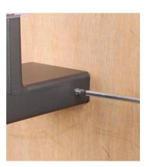
Using stents according to the picture above, nut on the screw holes and tighten
